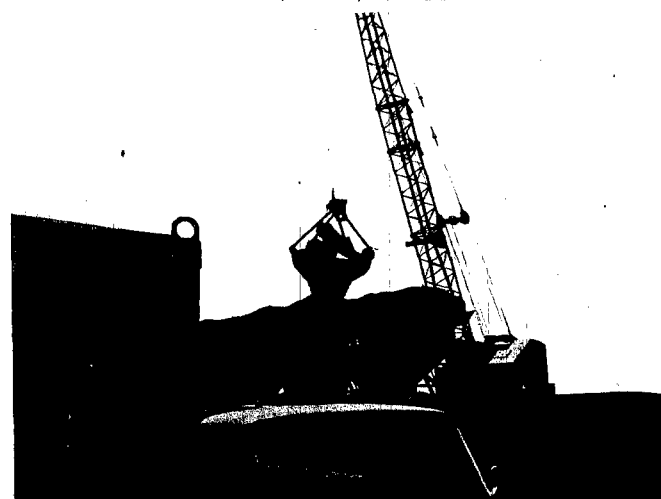
GIANT CRANE handles the big bucket with ease. Sand and gravel are transferred from ground into huge bins.
