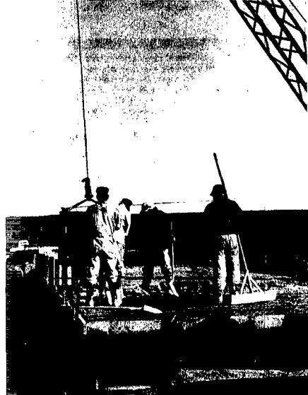
BRIDGE REPAIRING. These Dixon County workers were busy Thursday morning repairing the bridge about one mile north of Concord. The bridge collapsed September 12 when a heavy truck went over it. County workers estimated the work on the bridge would be completed sometime this week. The deck of the bridge will be six inches of concrete and should have no trouble supporting the heavy trucks in the future.
